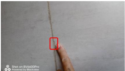
Paint splash marks on the finished tile.
