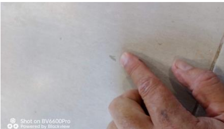
Paint splash marks on the finished tile.
