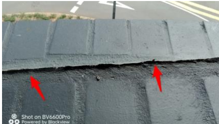
Balcony Guard Rail - Caulking substandard.
