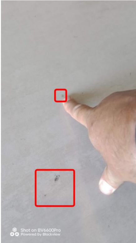
Paint splash marks on the finished tile.
