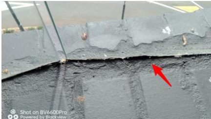
Balcony Guard Rail - Caulking substandard
