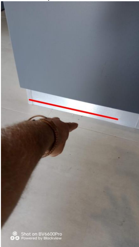
Kitchen kick-plate - seal off so no water damage occurs.
