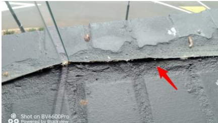
Balcony Guard Rail - Caulking substandard
