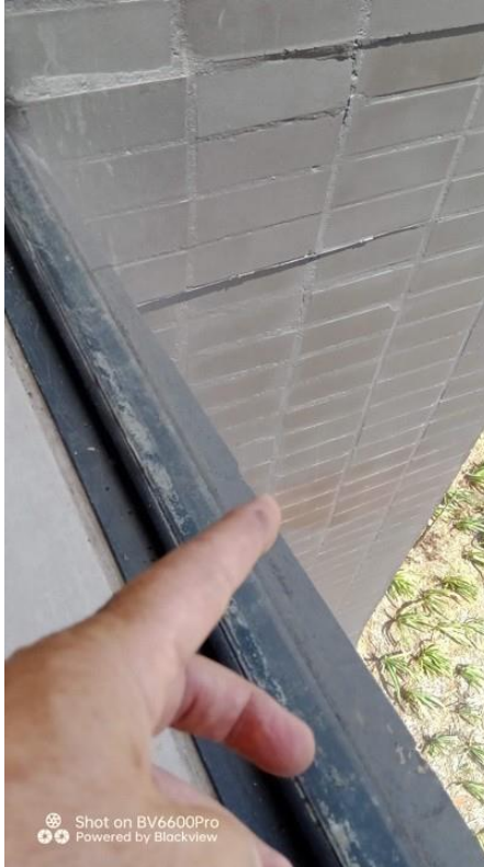
Scuff marks from building material on glazing.
