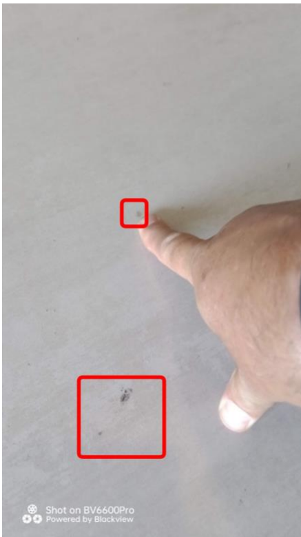
Paint splash marks on the finished tile.
