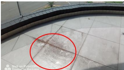
Ponding on a Tiled Balcony
