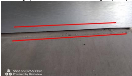
Kitchen kick-plate - seal off so no water damage occurs.
