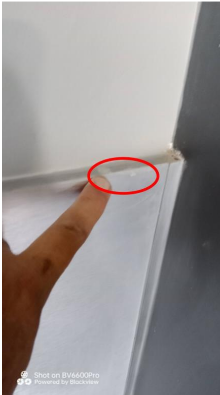
Paint spills on wall tile.
