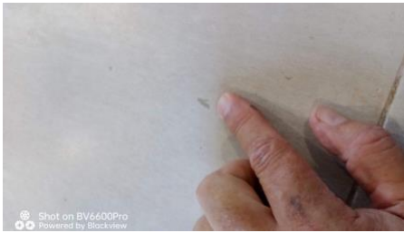
Paint splash marks on the finished tile.
