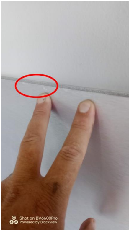
Paint spills on wall tile
