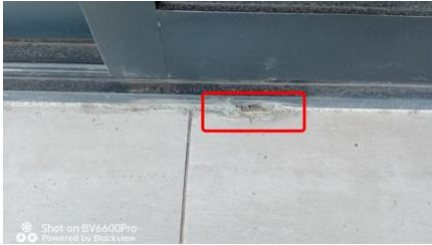
Balcony - grouting between tile and sliding door frame.
