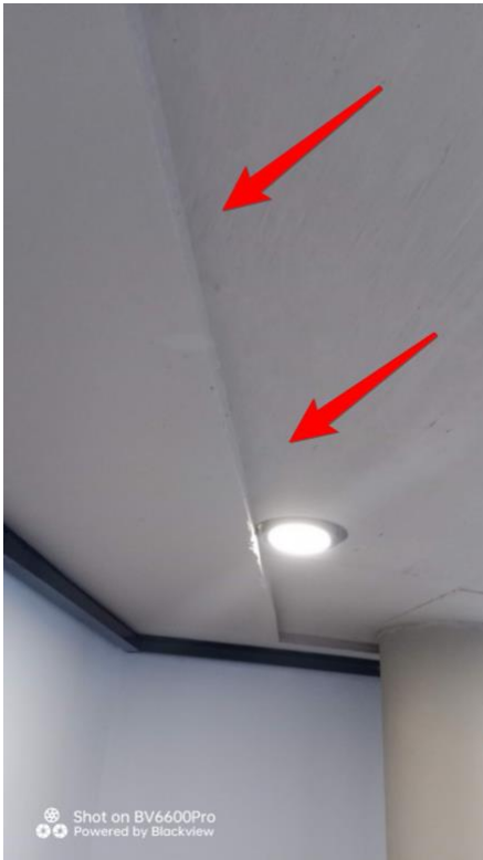
Stepped concrete ceiling
