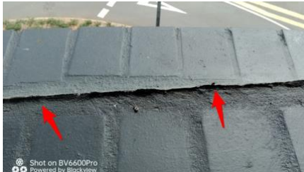
Balcony Guard Rail - Caulking substandard.
