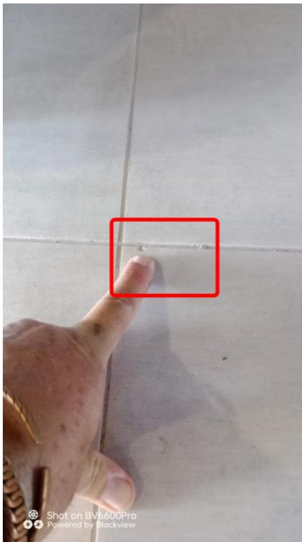
Paint splash marks on the finished tile.
